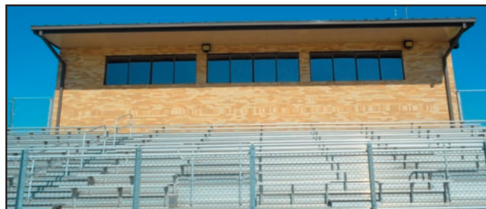
Track & Field Complex
